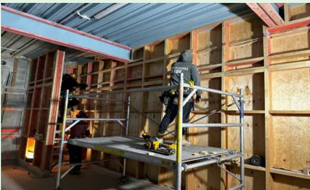
The Dawson Building crew working hard
